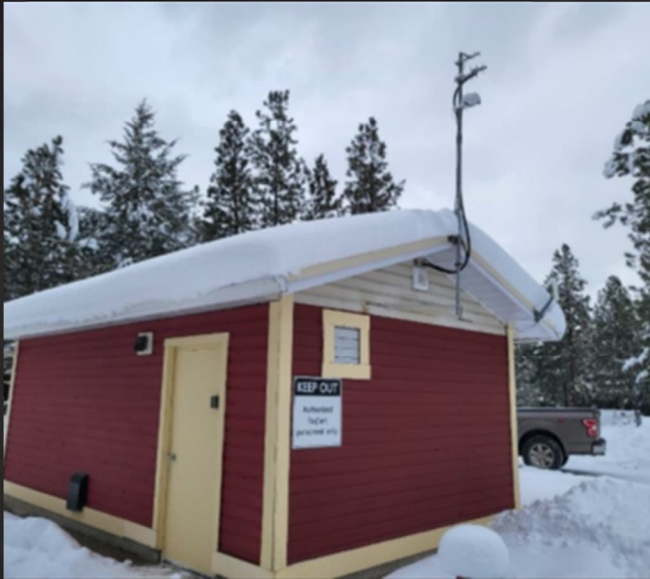
Figure 1: New Antenna installed for communicating pump and reservoir levels
